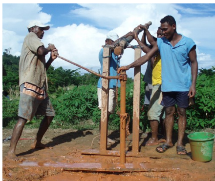
Manual drilling—Sludging
