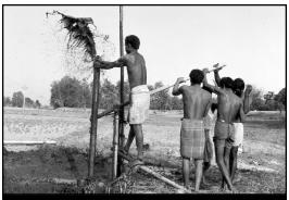
Figure 3 Drilling in progress for a shallow tube well
