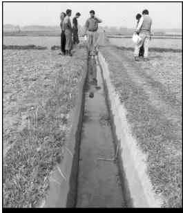
Figure 3 Soil-cement channel
