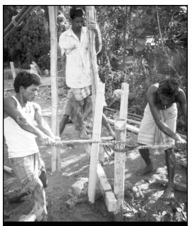
Figure 3 Back and forth movement of pipes
