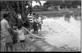
Figure 10 Jetting tool, using horizontal jets
