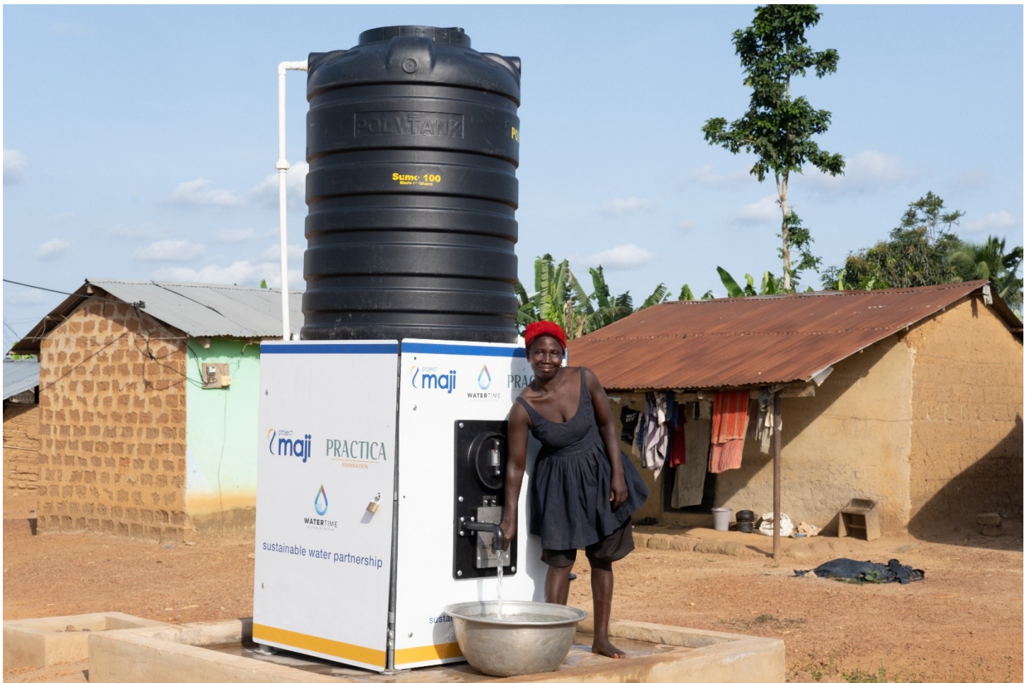
Photo: satellite tower in Ghana fitted with mechanical prepaid system. Source photo: Project Maji
