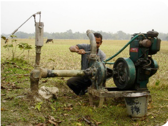
Figure 2 Indian diesel irrigation pumpset
