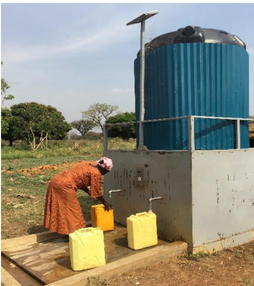
Figure 2 Satellite tower/ water kiosk that replaced handpump
