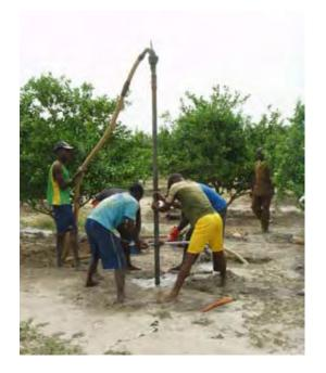
JETTING is based on water circulation and water pressure. As opposed to sludging, water is pumped down the drilling pipes. The large volume of water has an erosive effect at the bottom and the 'slurry' (water and cuttings) are transported up between the drill pipe and the borehole wall. A motor pump is used to achieve an adequate water flow. The drill pipe may simply have an open end, or a drill bit can be added and partial or full rotation of the drill pipe can be used.
