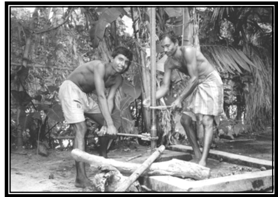
Figure 5.6; Gopal Adhikara and Sanjay Mishtri working for Nikhil Sarkar as labour mistris in hand sludge well boring
