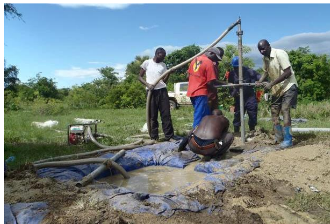
Photograph 1. Rotary well jetting in developmental context 3
