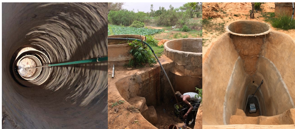
Figure 3 Unproductive deep well with a motor pump, motor pump and counter well, counter well
