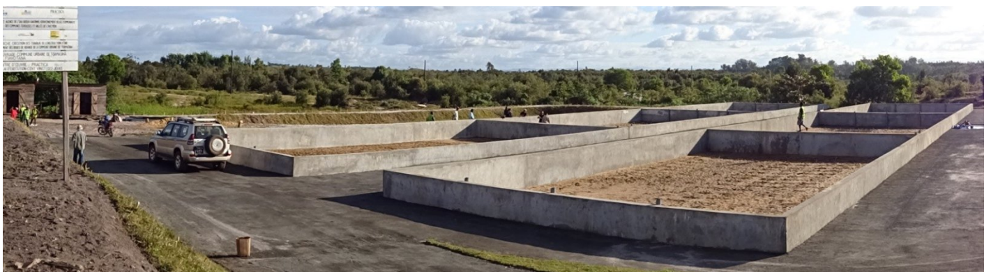
Fig.6 Fecal sludge humification plant in Toamasina (Madagascar) built by Protos and Practica (July 2016)
