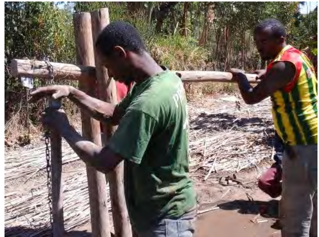
Figure 3: Drilling by the simple sludge technique
