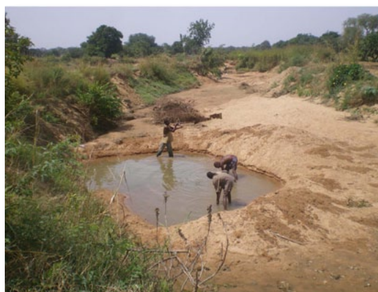
Figure 5: Alluvial Dugout under construction
