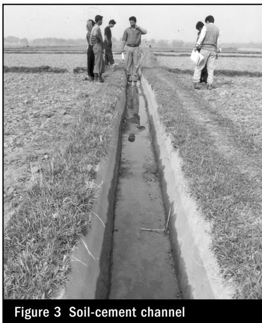
**Figure 3 Soil-cement channel**
