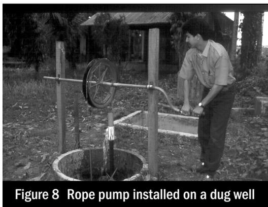
**Figure 8** Rope pump installed on a dug well
