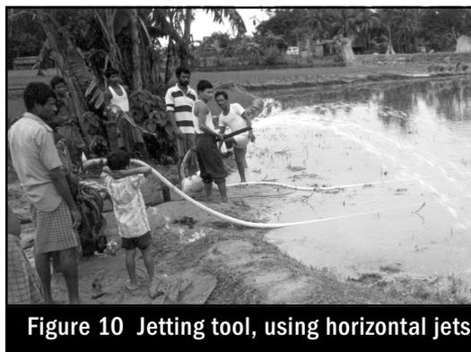
**Figure 10** Jetting tool, using horizontal jets
