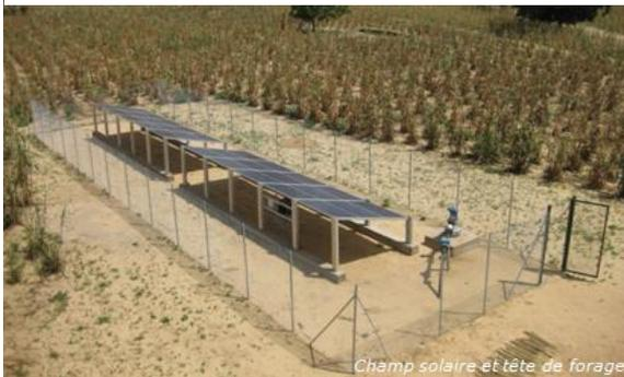
The other option is a plot on ground level, in the proximity of the borehole. The plot will need to be fenced, but it is anyhow necessary to fence the location of the borehole. But the fencing will need to be somewhat bigger and stronger. The advantages are that installation, maintenance, repair and cleaning are easier.
