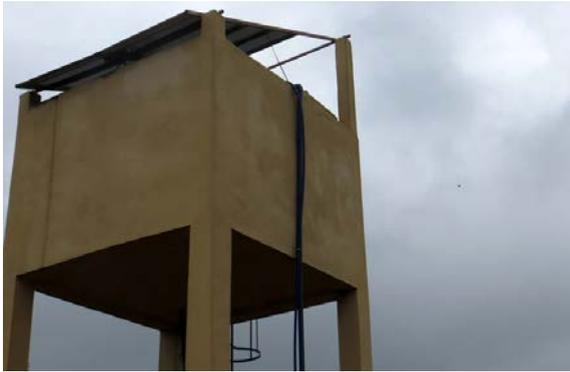
electric wires will be too long, which will bring along high electricity losses, or high costs for thick electric wiring to avoid these losses. The advantage of placing the array on the tower is that it is a good protection against theft of the panels. Moreover, the high place of the panels will also generally be a sunny place with little shadow, and the wind will cool down the panel easily.
